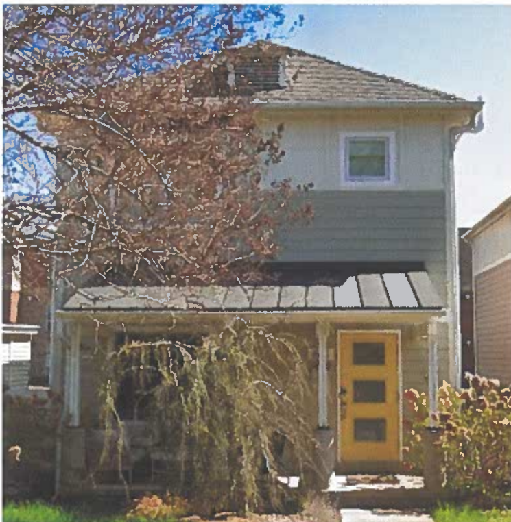
615 W. 19 th St. – Asphalt and Metal
