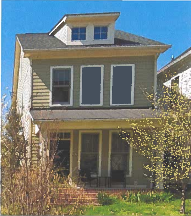
506 W. 19 th St. - Asphalt and Metal
