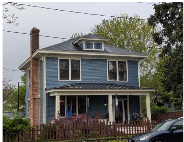
Figure 2. Existing condition of 510 West 20th Street.
