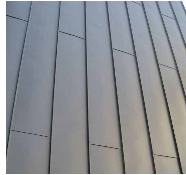
ZINC STANDING SEAM ROOF
