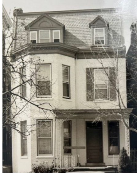
Figure 2. 1809 West Grace Street, 1977, HRF Survey. Original front porch has been removed and replaced with mid-century, decorative metal posts and railings. Original entablature appears to be in place. Building has been painted.
