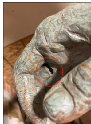
B. Crack detail
