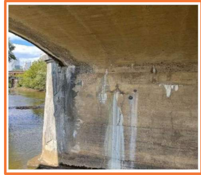
Figure 4a from Sub-structure Analysis Report: Grout leak through pier wall
