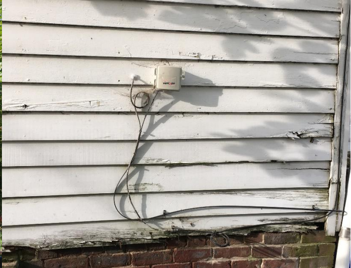
Figure 4. Rotted wooden siding
