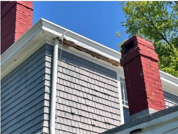
Figure 3. 4002 Hermitage, existing conditions, built-in gutter deterioration
