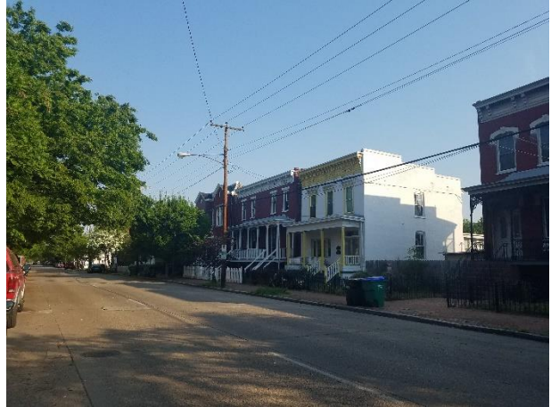
Figure 2. View west along West Clay Street towards 128 W. Clay.
