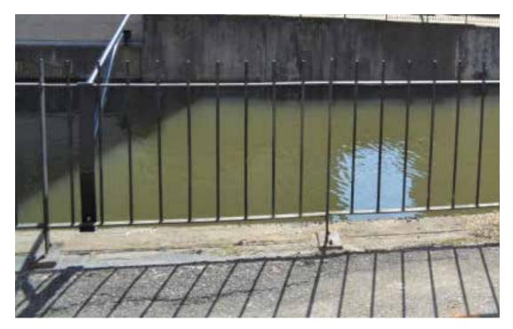
METAL RAILINGS ALONG CANAL EDGE FOR SAFETY - REPURPOSE OR MATCH EXISTING ADJACENT METAL CANAL RAILINGS
