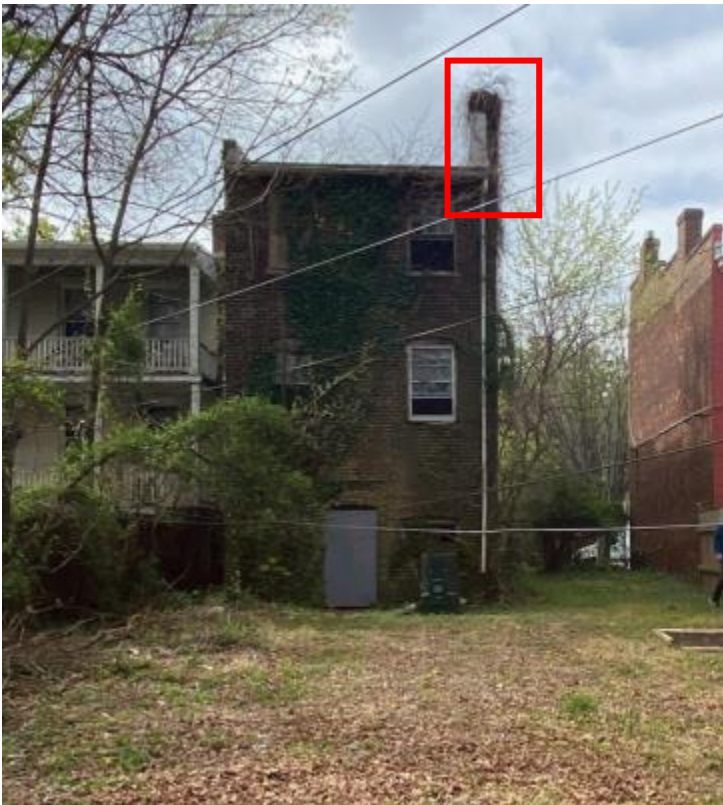
Figure 3. Rear elevation of 2320 East Marshall St.
