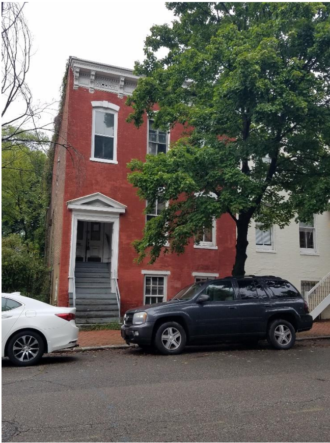
Figure 1. Façade of 2320 East Marshall Street
