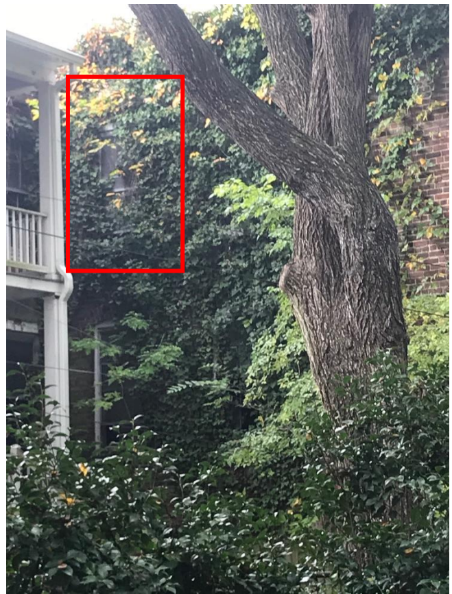
Figure 2. View of side elevation from North 24th Street.
