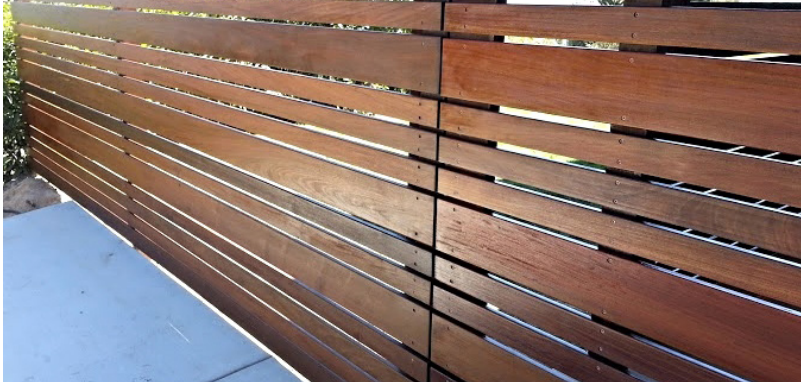
Alternating 1x6 & 1x3 Cumaru Fencing w/4x4 P.T. Post Pntd.
