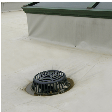
Internal Concealed Drainage System
