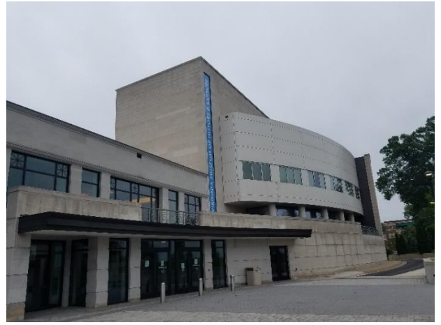
Figure 2. South (VMFA facing) elevation. Proposed changes include enclosing the curved section, removal of the east railing and in-filling the space with masonry, and removal of the west railing and installation of glass panels.
