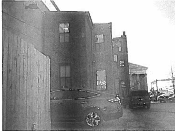
Figure 2: 18 West Franklin, rear view
