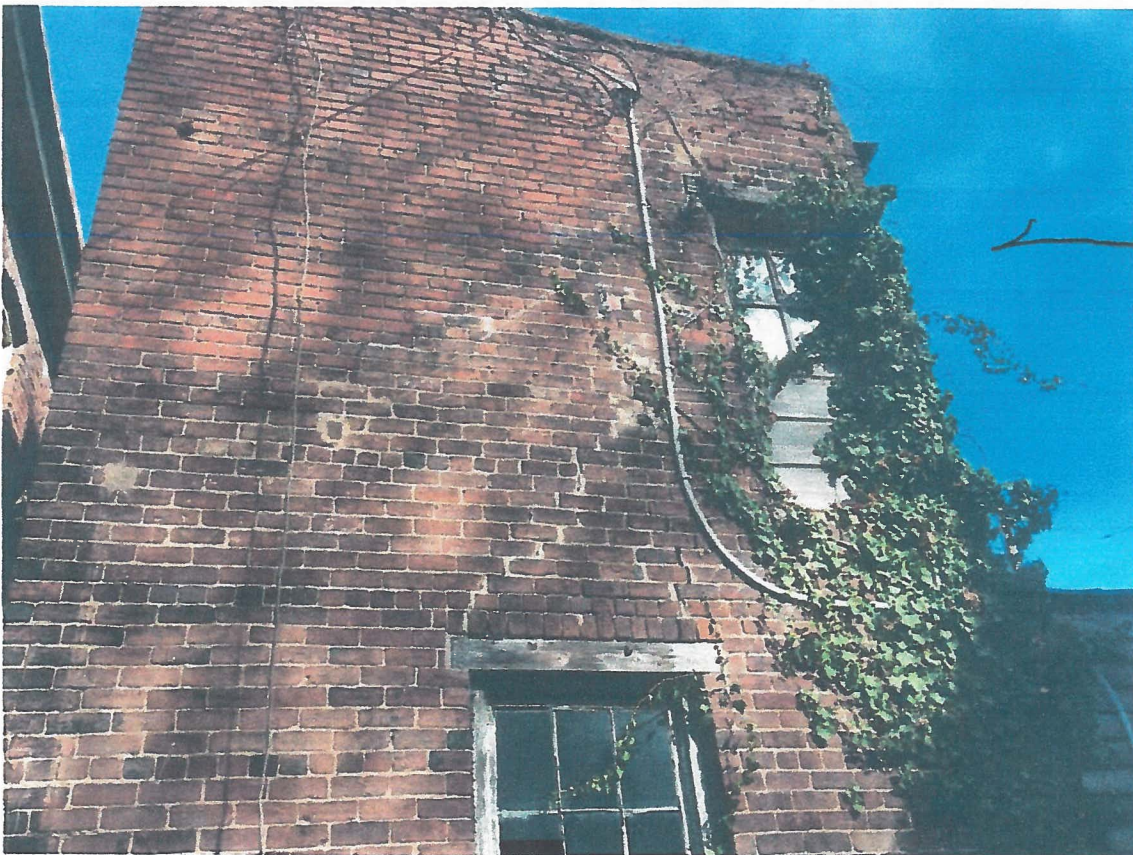
8. Rear elevation, looking north. Note structural cracks and top corner of parapet where bricks are caving in and falling out
