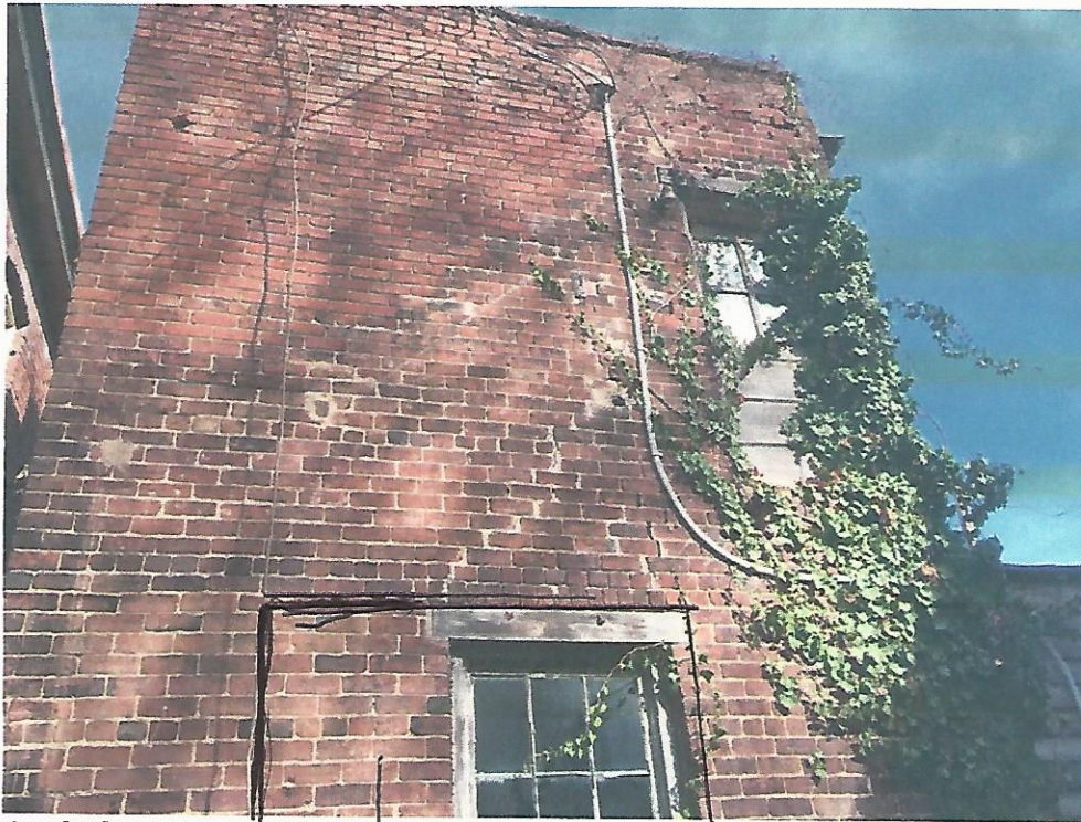
8. Rear elevation, looking north. Note structural cracks and top corner of parapet where bricks are caving in and falling out
