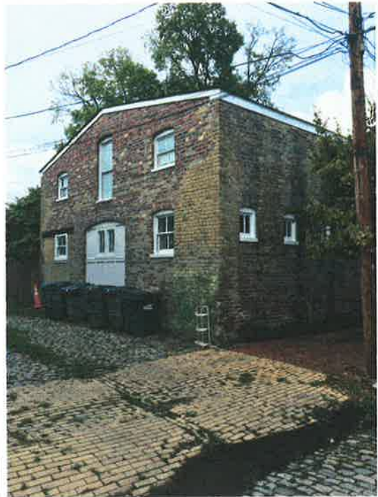
Examples of square windows at 2623 East Broad Street; side windows have single vertical mullion
