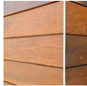
SHIPLAP WOOD SIDING: CEDAR OR SIMILAR SPECIES WITH CLEAR PROTECTIVE FINISH
