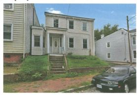
The above picture shows there is an existing "addition" to the home on the left side. It is attached directly to the neighboring house. The below picture shows the improper construction of the roof from above. The improper design of the bump out and the improper roof installation has caused this area to flood and destroy the structural framing. We are proposing to remove the structure and "detach" the 2 homes. The below picture to the right shows the original siding on the neighboring home.
