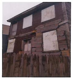
Brick in front of structure to remain as is - all existing damaged material (wood and roofing substance used as siding material) to be removed.
