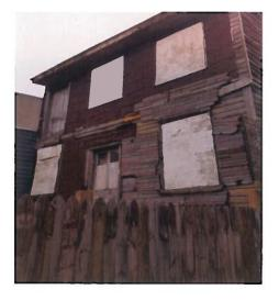
Existing 3 damaged doors to be removed. Rear top entryway to be removed - leaving one lower-level doorway in front and one lower-level doorway in rear. Doors will be replaced with Masonite 6-Panel Solid Wood Core Hem Fir Unfinished Slab Entry Door and painted 41 - Classic Light Buff, SW #0050, RGB (239, 236, 221). Hardware to be replaced Kwikset Arlington Adjustable Antique Nickel Entry Door Exterior Handle.
