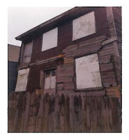
Windows to be restored - all window glasswork should still be intact. Damaged framework to be replaced - reconstruction to be done using wood and painted 41 - Classic Light Buff, SW #0050, RGB (239, 236, 221)
