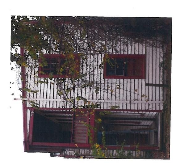
Excessive vegetation (vines and brush) have held moisture against the siding, leading to water damage.
