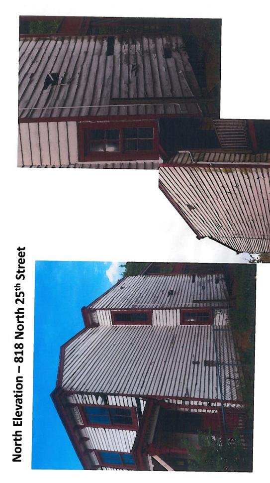
The north elevation has the most damage due to moisture, warped boards and broken boards.
