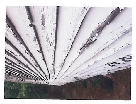
The southside of the home receives intense sun and wind exposure. Due to the lack of maintenance over the years, a significant portion of the boards are rotted and beyond repair. Contractor estimates indicate that the entire southside will need to be replaced and is beyond repair.
