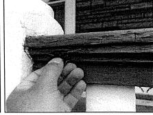
There were many instances of rot observed at the second floor porch including decking boards, wood trim, the main posts, and in the eaves above the main posts. I recommend repair by a qualified contractor. (\$500-\$800+)
