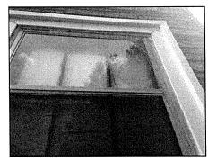
The rear exterior window had a crack in the pane. This was not observed from the interior due to the addition of the downstairs shower. I recommend repair by a qualified glazier or contractor.
