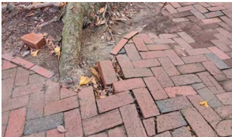
Uprooted brick pavers from tree roots
