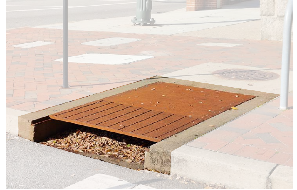
Corten steel is used for storm drains to offer a unique aesthetic to the streetscape.
