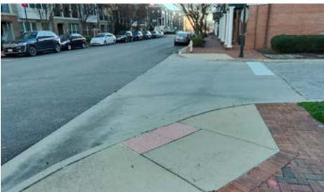
Pedestrian ramps are concrete ramps, with concrete aprons
