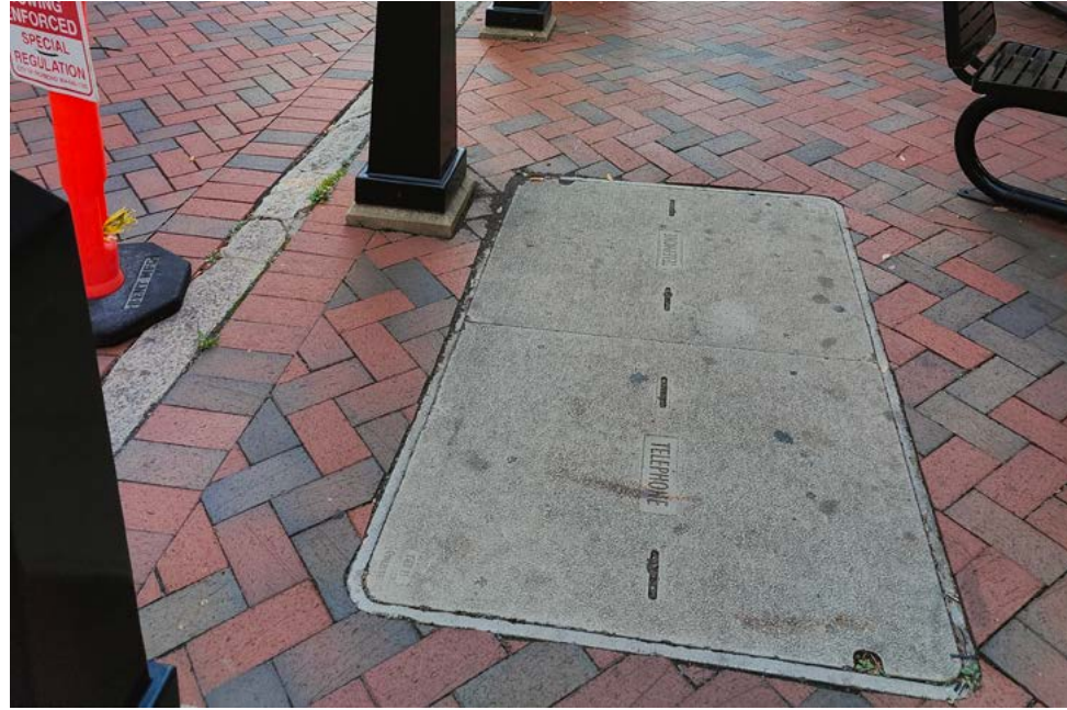
Manholes and utilities are located in the center of the sidewalks for quick access, but do not blend with the surrounding materials.
