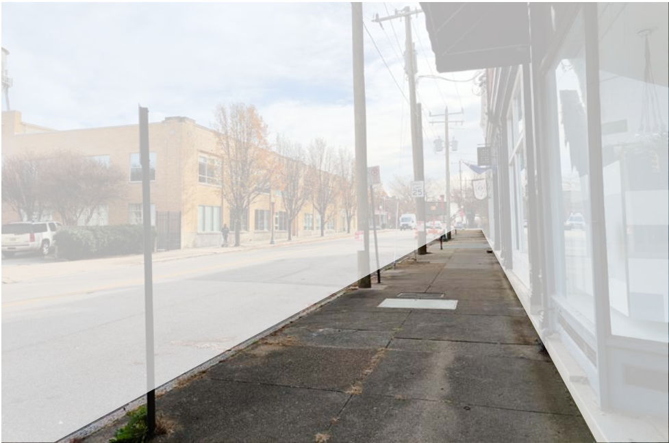
A lack of maintenance has caused Church Hill sidewalks to have cracks, moss, and weed growth.
