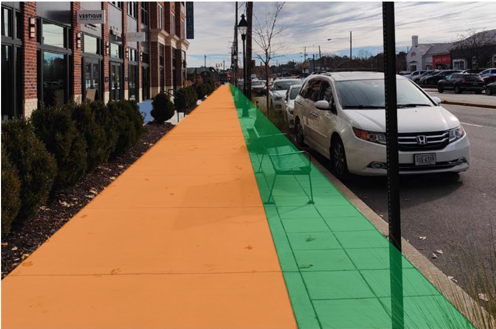
All three sidewalk zones are clearly distinguish through the use of furnishings, planting, and a change in concrete scoring.
