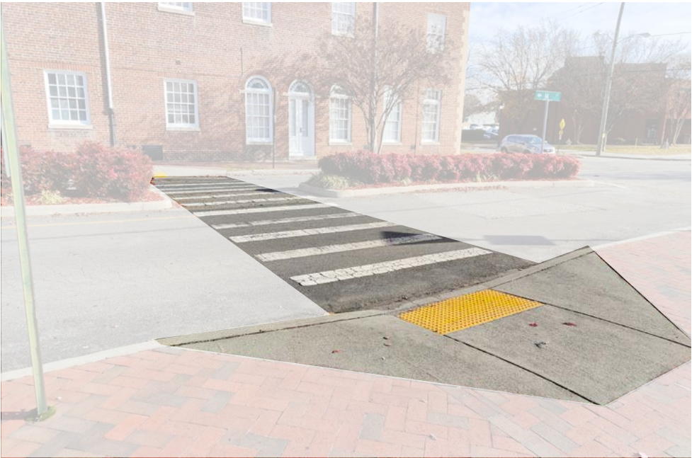
Pedestrian crossings are currently a CG-12 ramp and white block style painted asphalt.
