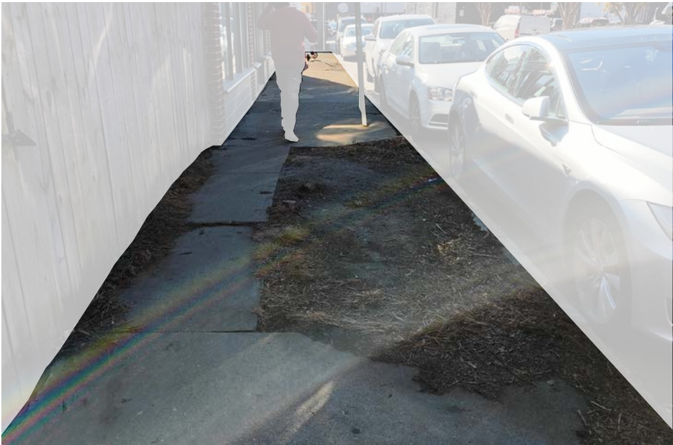
Poor maintenance has resulted in spreading mulch beds, cracked mossy sidewalks, and weed growth.
