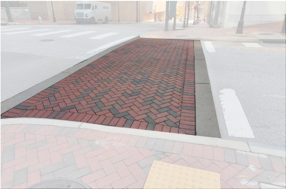
Pedestrian crossings include a concrete border and a herringbone brick paver pattern.
