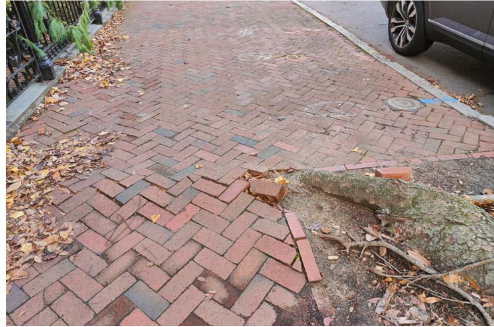
A lack of maintenance has caused tripping hazards and a poor surface for wheelchair users.
