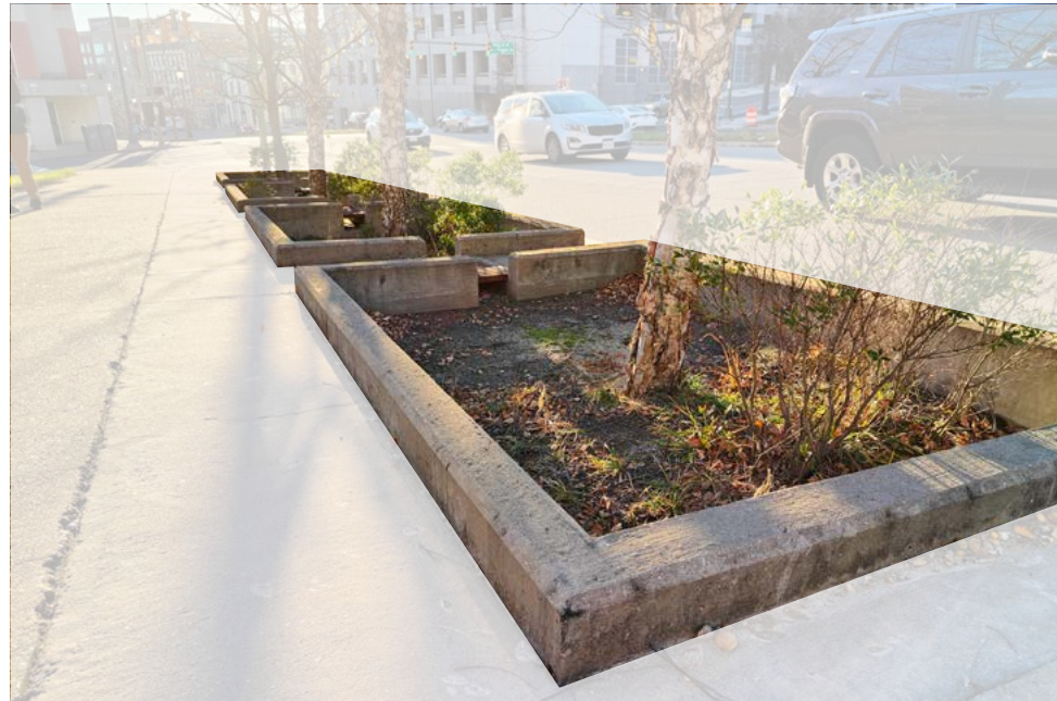
Tree wells located along 14th street are designed for stormwater capture, yet poor design and maintenance results in dangerous element for pedestrian users.
