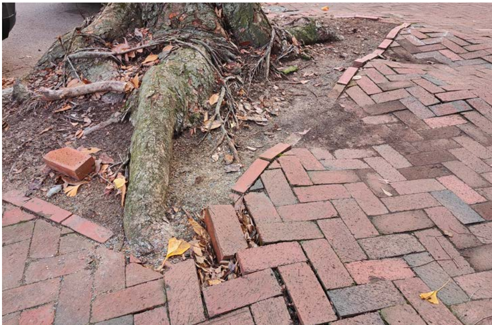
Larger, historic trees have caused the existing pavers to move do to the growth of the tree root system.
