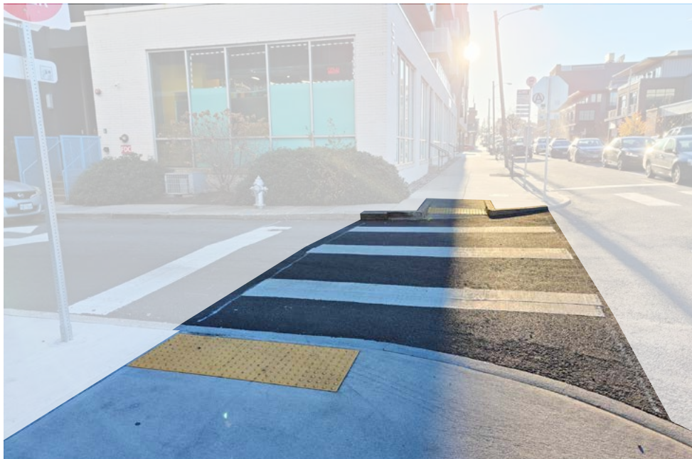
Pedestrian crossings are white block styles with lowered detectable warnings for all site users.
