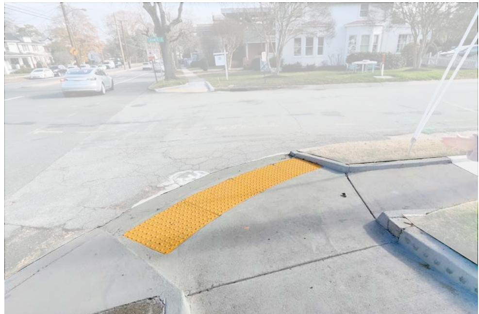
CG-12 ramp located at existing intersections.
