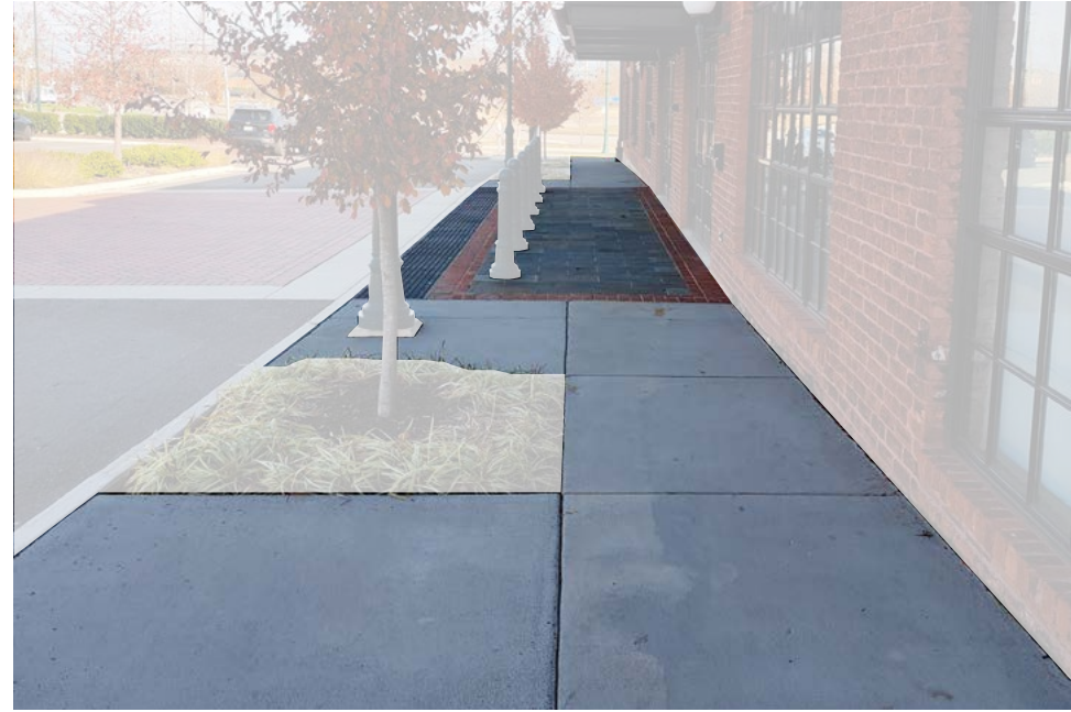
Sidewalks are predominantly scored concrete, with a change of material to reflect a point of interest.
