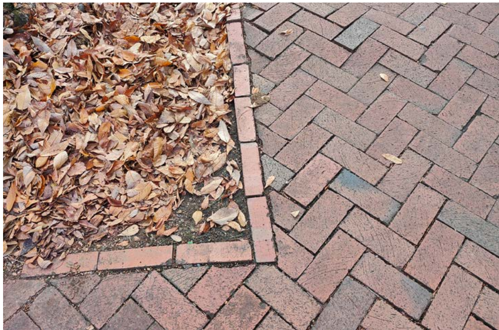
Brick pavers are used in multiple places throughout the streets, including borders, accent bands, and main thoroughfare routes.
