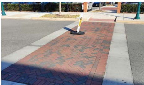
Brick pavers with a herringbone pattern and concrete border
