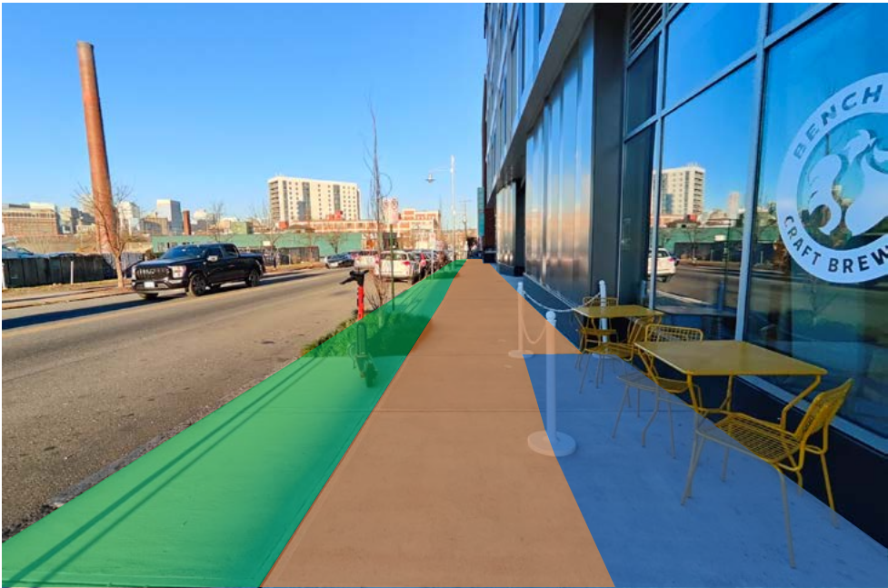
No changes in sidewalk material or score pattern makes it difficult to distinguish between the Frontage Zone (blue) and the Pedestrian Travel Zone (orange).
