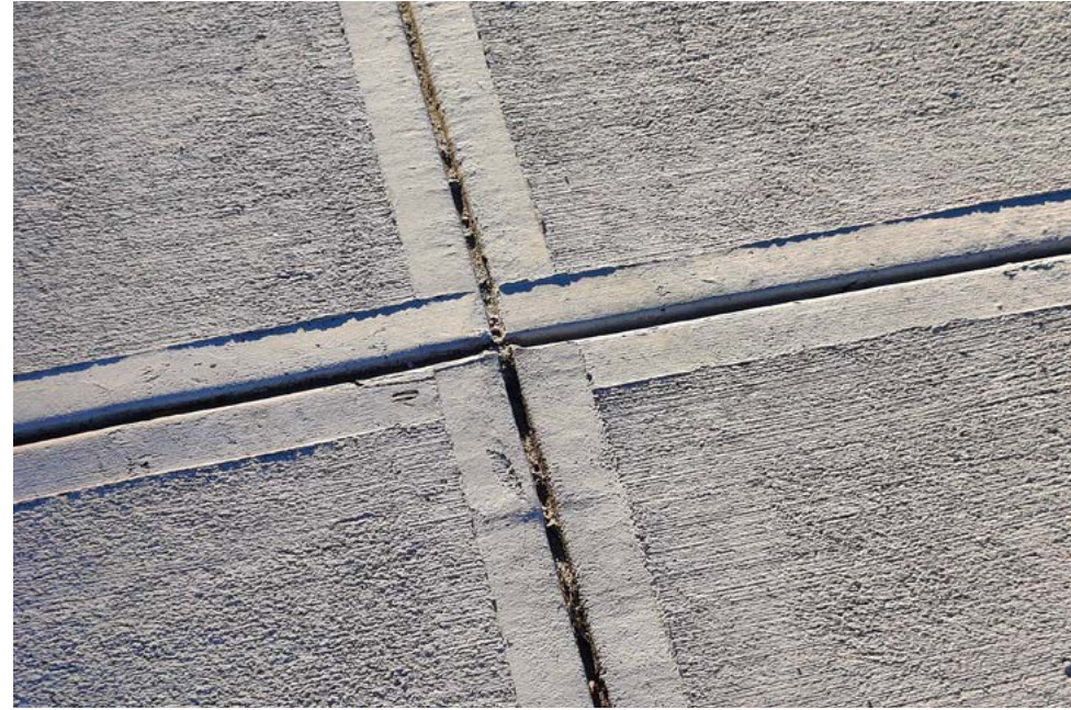
Concrete scores lines are constructed with a flat border for visual variety throughout the development.
