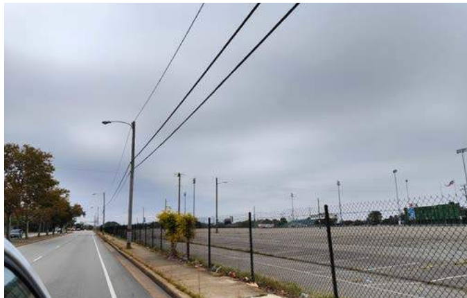
Overhead power lines shall be located underground
