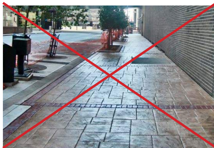
Dyed and/or stamped concrete is not permitted.
