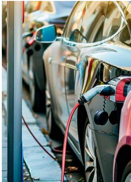
EV Charging Station
