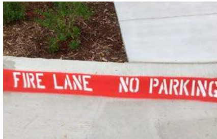
Fire Lane Markings
