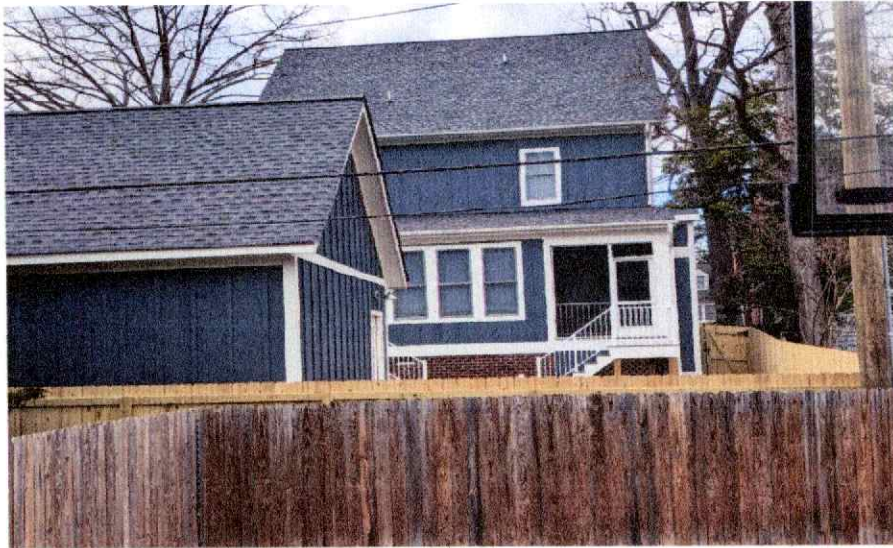
Note the interior fence in the foreground as it corners to the left---this shows how the Garage covers more than one-half (within the side yard setbacks) of the total span of the lot
