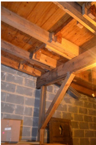
Figure 9. Interior view of the garage's east wall. The photograph shows additional wall braces added to support the unsound roof.
