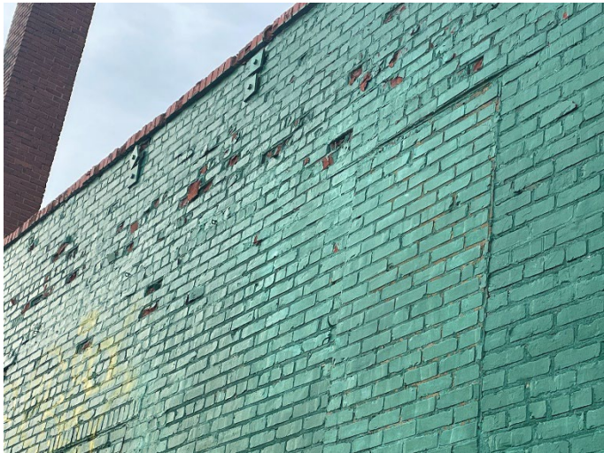
Figure 8. Brick Spalling example.
