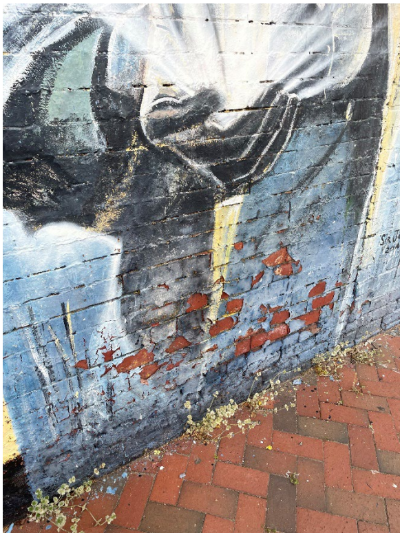
Figure 7. Brick Spalling/ Up splash causing paint deterioration example.
