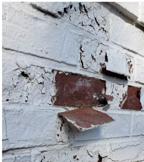
Figure 4. Brick Spalling example
