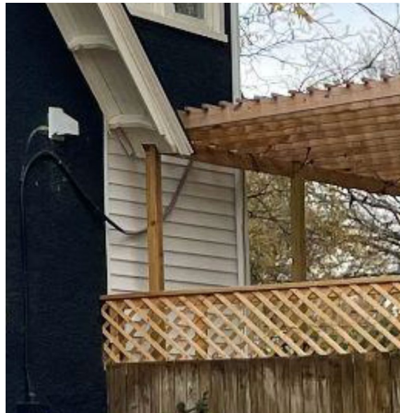
Figure 4. Notch cut into existing eave to accommodate pergola.
