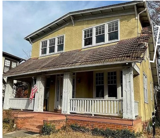
Figure 2. Deteriorated Concrete Tile Roof, 3833 Hermitage Road. Before
