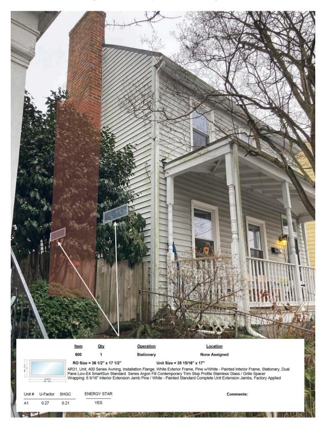
Addition of one bedroom window on the east elevation. Andersen, wood, no divided lights. Same trim style/width as existing. Same size as existing window. Replacement slider from 6ft to 8ft. Andersen, wood, no divided lights. Same trim style/width as existing.
