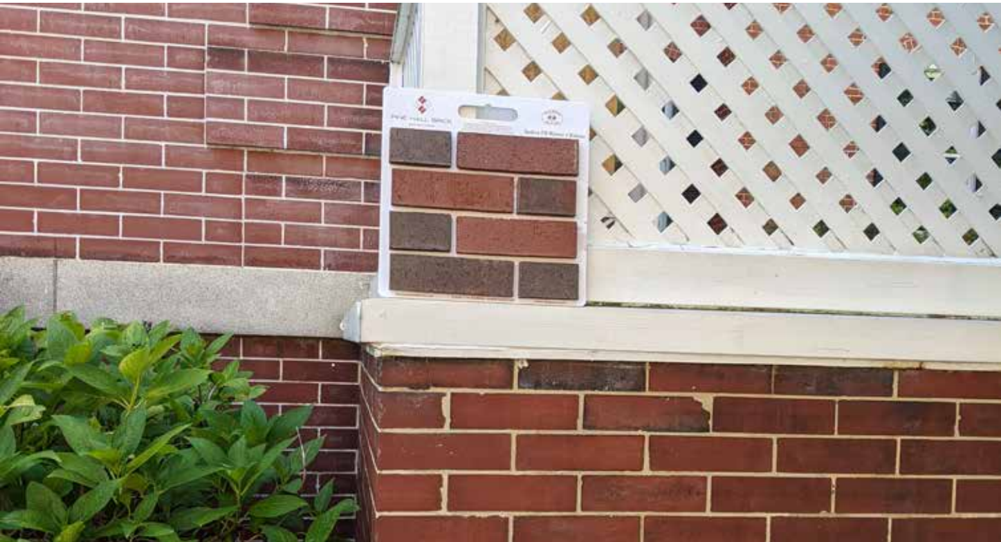
AS THE WALL ROUNDS THE CORNER AND CONNECTS TO THE HOUSE DARKER GRAY BRICKS WILL BE REMOVED FROM THE MIX TO MAKE A NICE TRANSITION TO THE HOUSE (WHICH DOESN'T HAVE A VARIED COLOR RANGE, BUT APPEARS TO BE MADE OF THE SAME BRICKS USING JUST RED)
