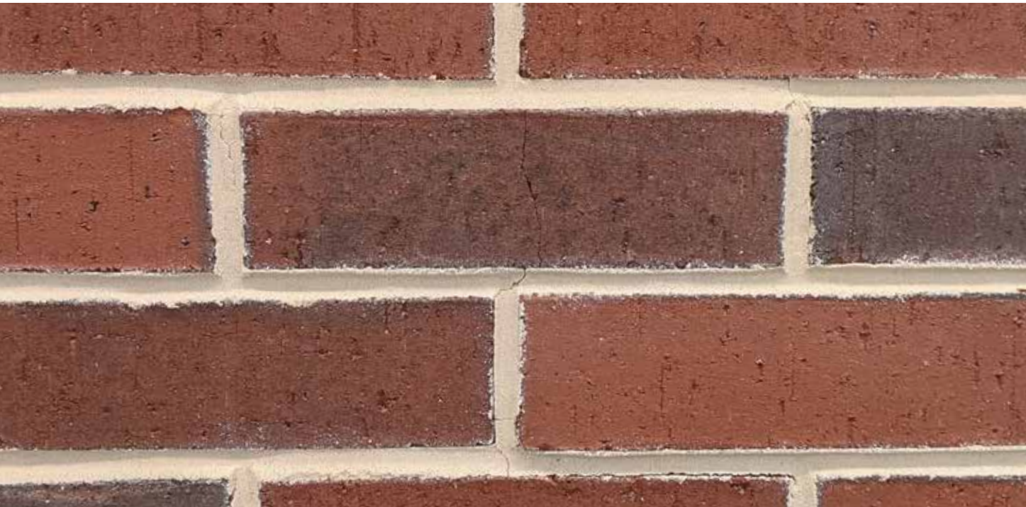
MORTAR - ARGOS 'SAHARA' COLOR, WITH A SLIGHTLY WIDER JOINT THAN EXISTING WALL SHOWN WITH ACTUAL BRICK SPECIFICATION
