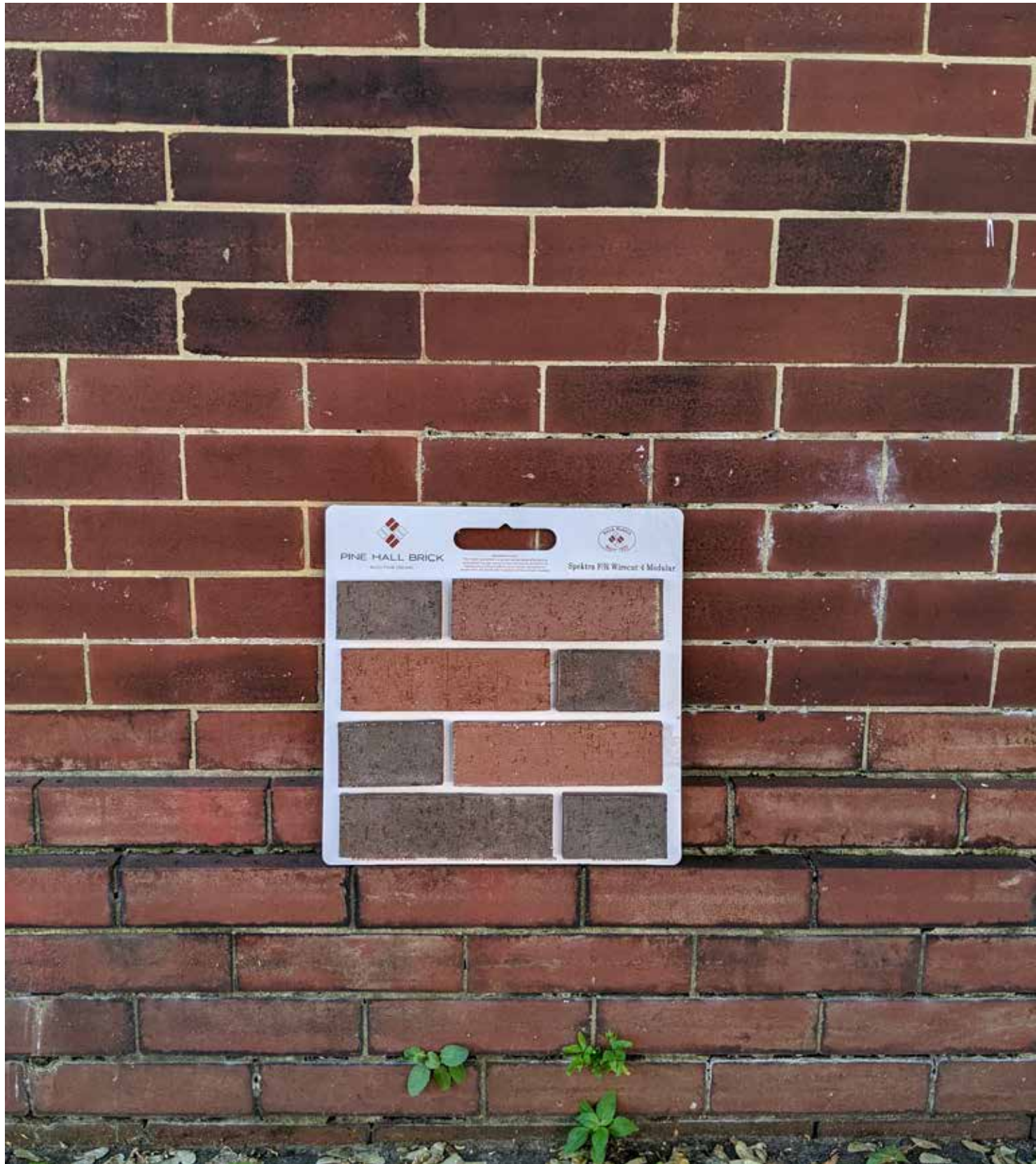
BRICK SELECTION - MODULAR WITH A LIGHT WIRE CUT TEXTURE (EXISTING BRICK ARE SMOOTH) PINE HALL BRICK - SPEKTRA FULL RANGE
