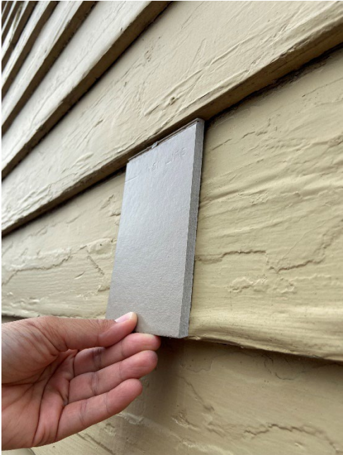
Fiber cement, HardiPlank, comparison to existing wood siding.
