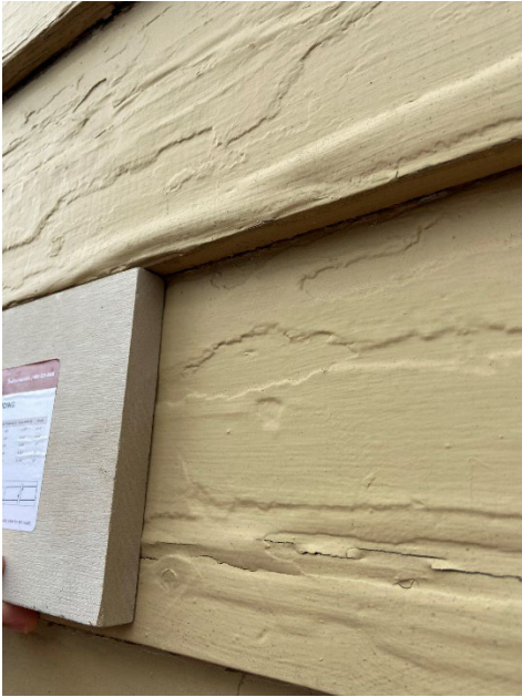
Boral comparison to existing wood siding
