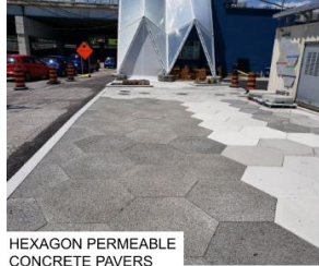
HEXAGON PERMEABLE CONCRETE PAVERS
