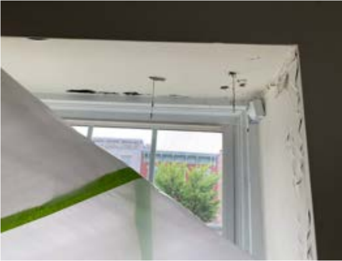
Figure 4. Interior water damage and mold
