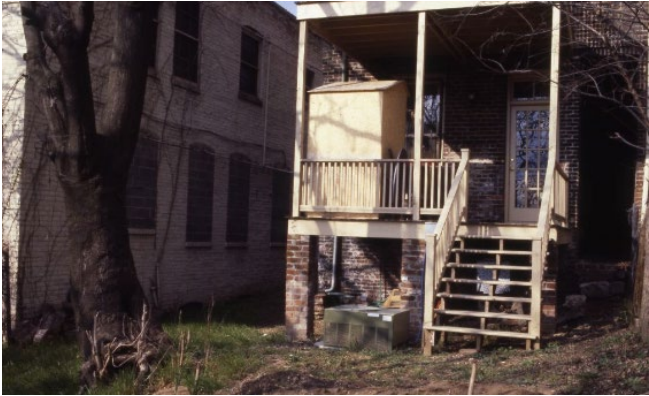
Figure 4. Original rear porch design at attached 2509 E. Franklin Street. Simple design with slim square posts and Richmond Rail.
