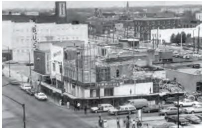
Construction of Covention Center
