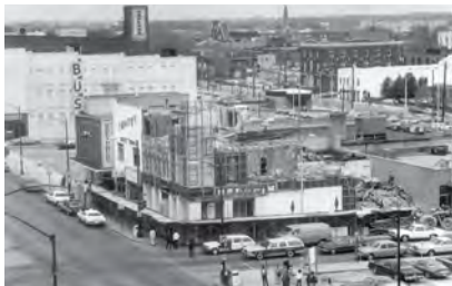
Construction of Covention Center
