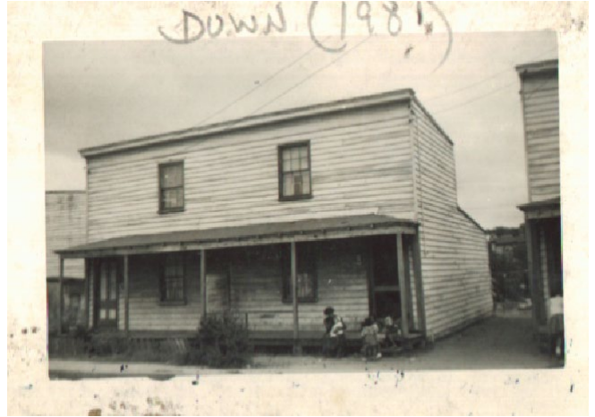
Figure 2. Historic image of original structure on the subject parcel. Demolished 1981
