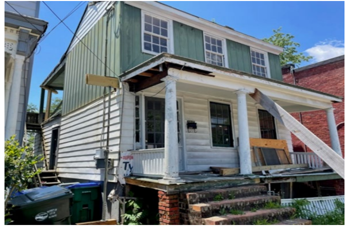
Figure 2. Front and East façade photo
