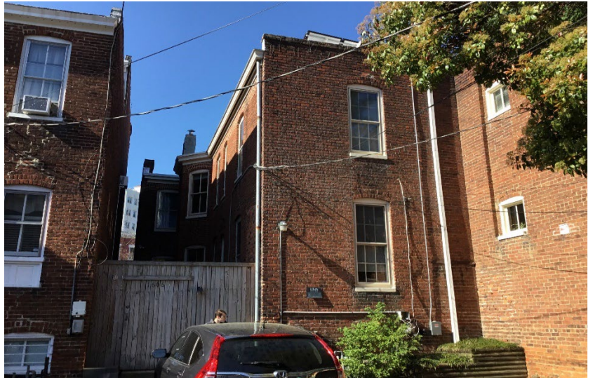
Figure 2. View of rear façade, existing.
