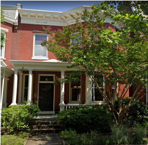
Figure 1. Front façade, existing.
