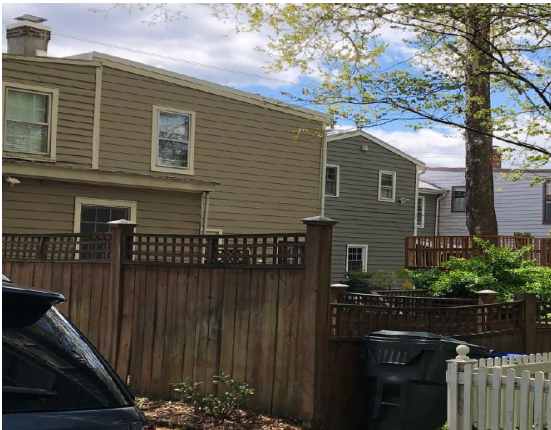
Figure 3. View of rear seen from N. 27 th Street
