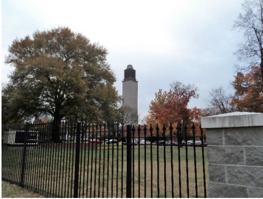
Figure 2. Belgian Building belfry, November 2019.
