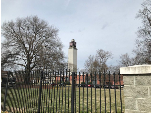
Figure 2. Belgian Building belfry, current conditions.
