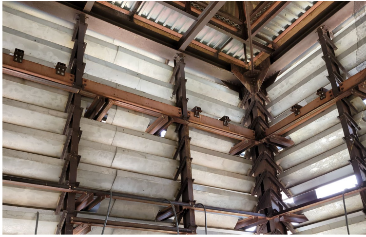
Figure 5. Sign connection to the bell tower, as shown from the interior.
