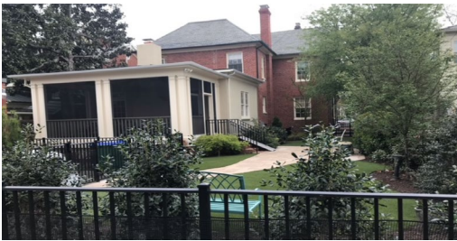
Figure 3. Existing rear aluminum fence. CAR Files, Feb. 2019
