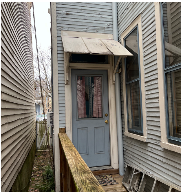
Example of bracketed roof overhang at side door
