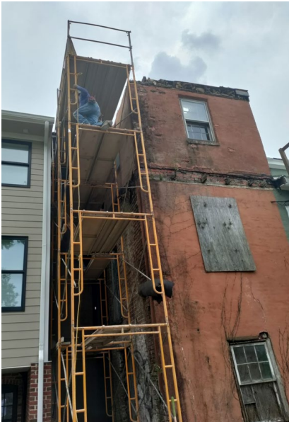
Figure 3. Photo from before August 2021 showing the poor condition of the rear wall before demolition
