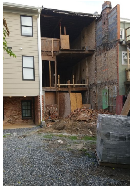
Figure 4. Photo from August 2021 showing the post-demolition rear wall
