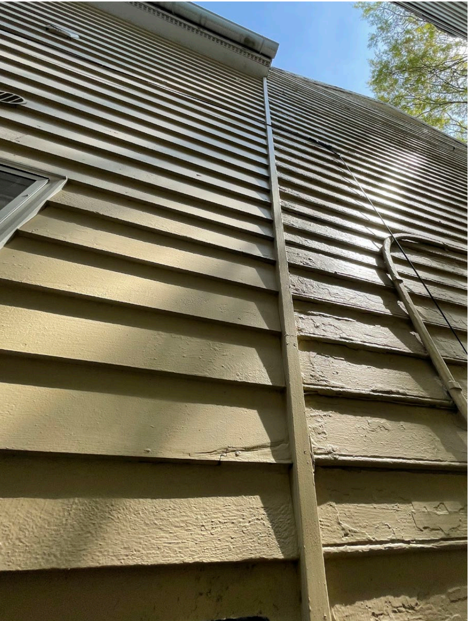
EXISTING SIDING DETAILS – A TWO-STORY VERTICAL BATTEN TRANSITIONS FROM THE OLDEST HISTORIC SIDING (RIGHT) TO EXISTING SIDING AT A PREVIOUS ADDITION (LEFT) THE OLDEST SIDING CONSISTS OF BEADED SHIP-LAP WHILE NEWER SIDING MATCHES THE TYPICAL HISTORIC EXPOSURE HEIGHT BUT WITHOUT THE HISTORIC BEAD. A SIMILAR APPROACH WILL BE TAKEN FOR NEW SIDING ELEMENTS.
