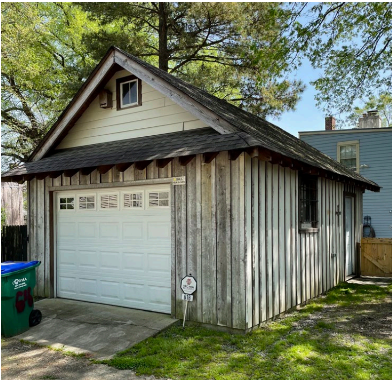
REAR ALLEY AT 616 N. 27th STREET – BATTEN SIDING W/ EXPOSED RAFTERS
