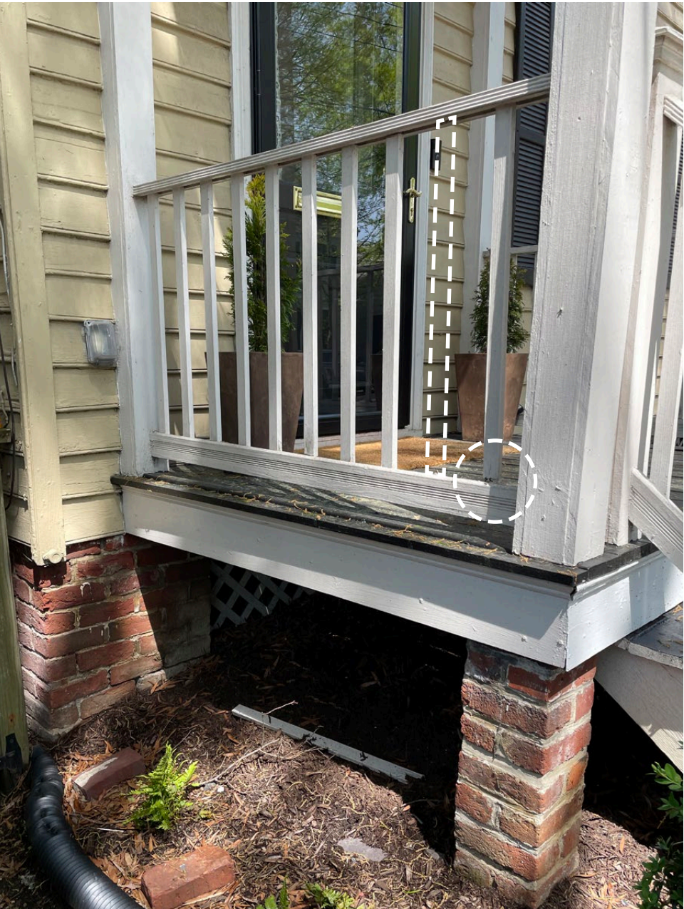
EXISTING FRONT PORCH SHOWING TYPICAL PICKETS TO BE REPAIRED / REPLACED IN KIND
