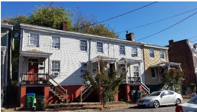
Figure 5. 521-527 N. 24th Street
