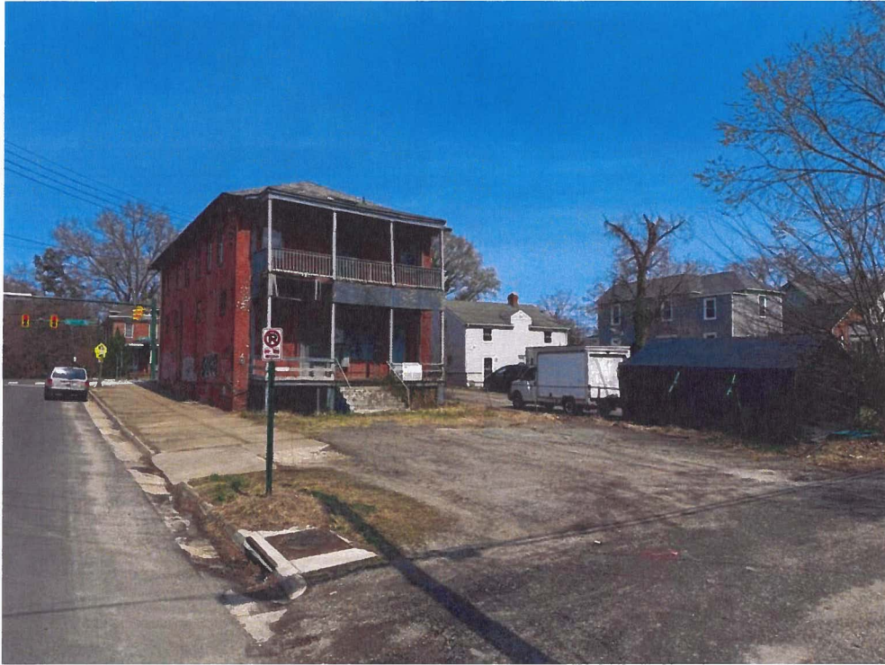
Rear Elevation - note alley access, curb cut, & ample off-street parking
