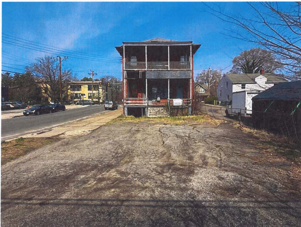
Rear Elevation – note dedicated access to the commercial space via door at left and private access to a 1BR apartment on second floor via door at right
