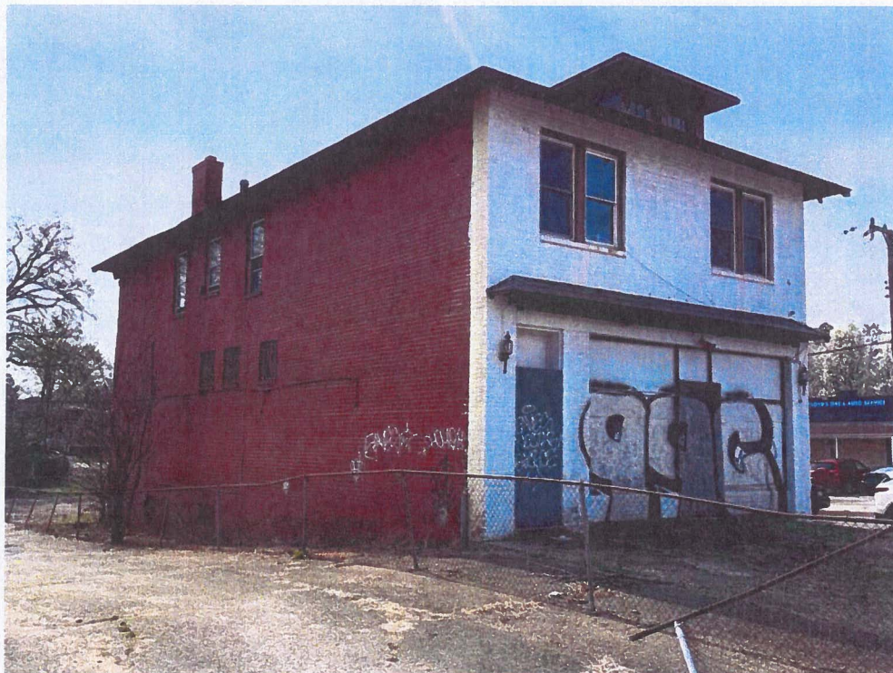
East Side Elevation – note access to rear parking along left side
