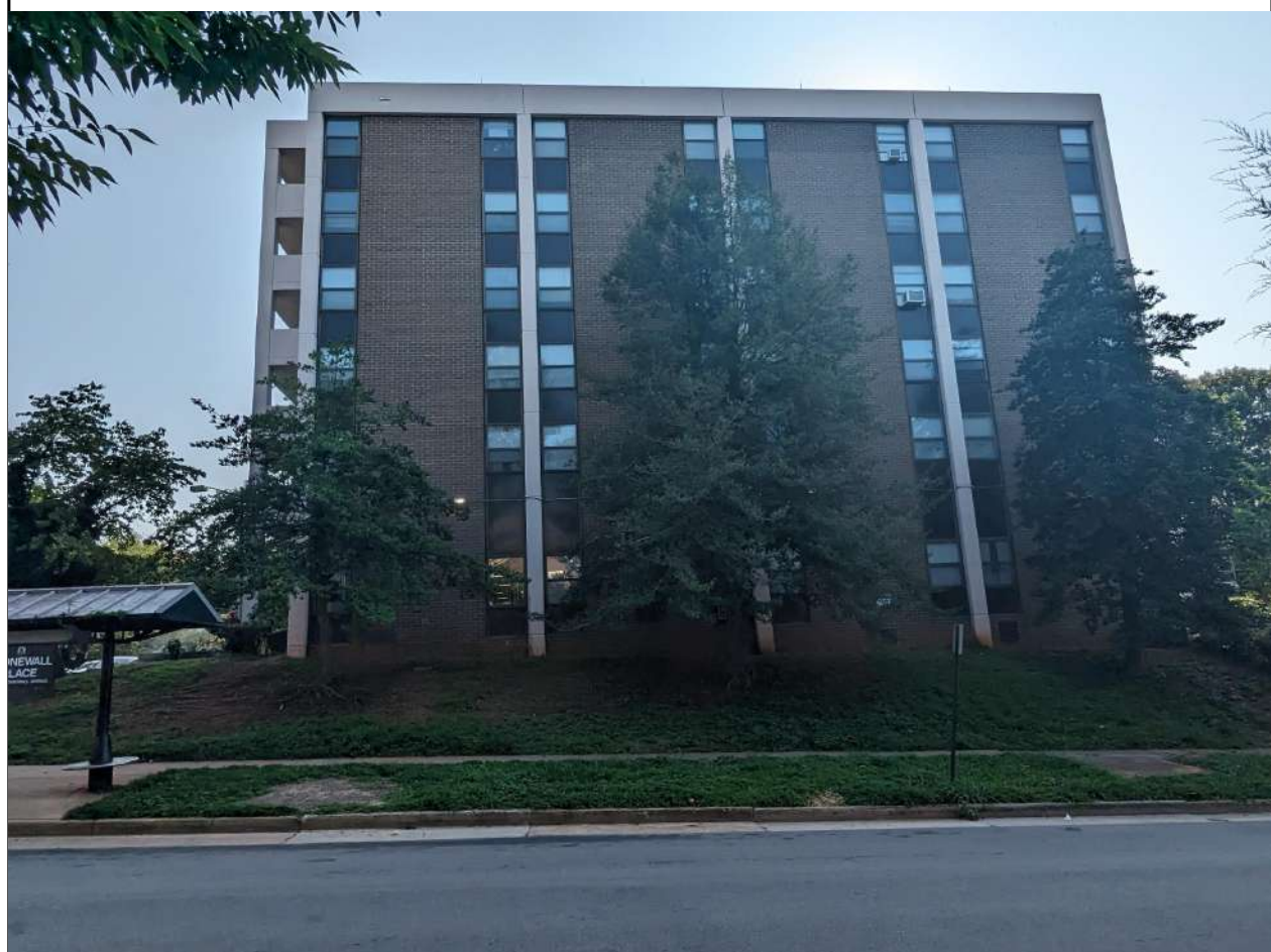
BUILDING DIRECTLY ACROSS W. 20TH STREET
