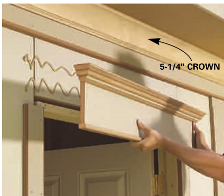
11 Nail and glue the moldings to the frieze board one at a time. Then fasten the head casing above the door with construction adhesive and brad nails.
