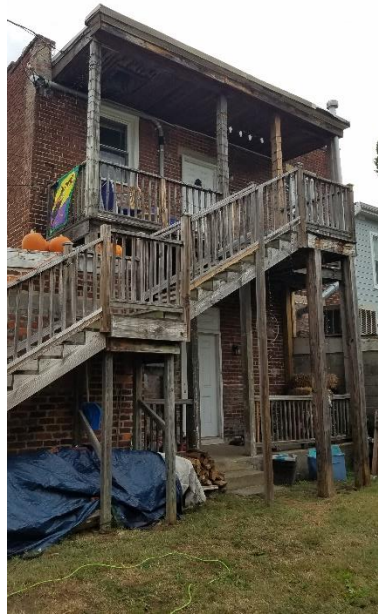
Figure 6. 3105 East Marshall Street, rear elevation.
