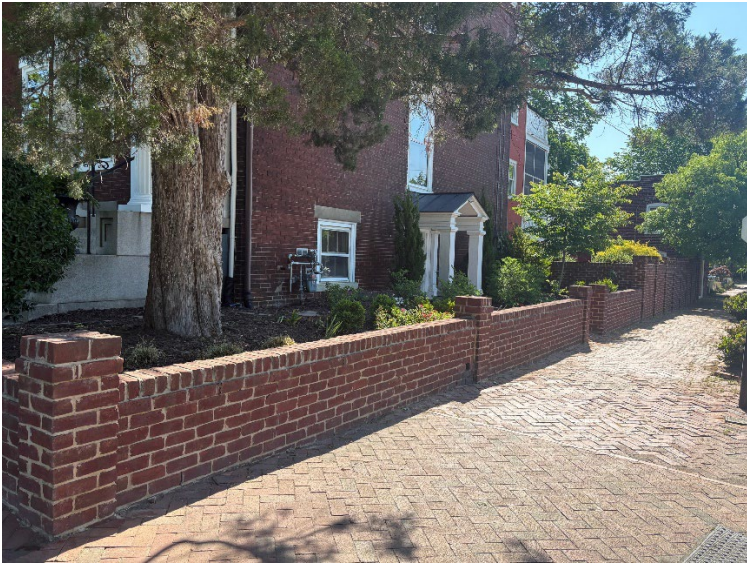
Figure 5. . Example of new brick wall approved by CAR in 2022. April 2026.
