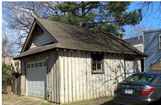
Figure 5. Outbuilding Example Located on the Same Block
